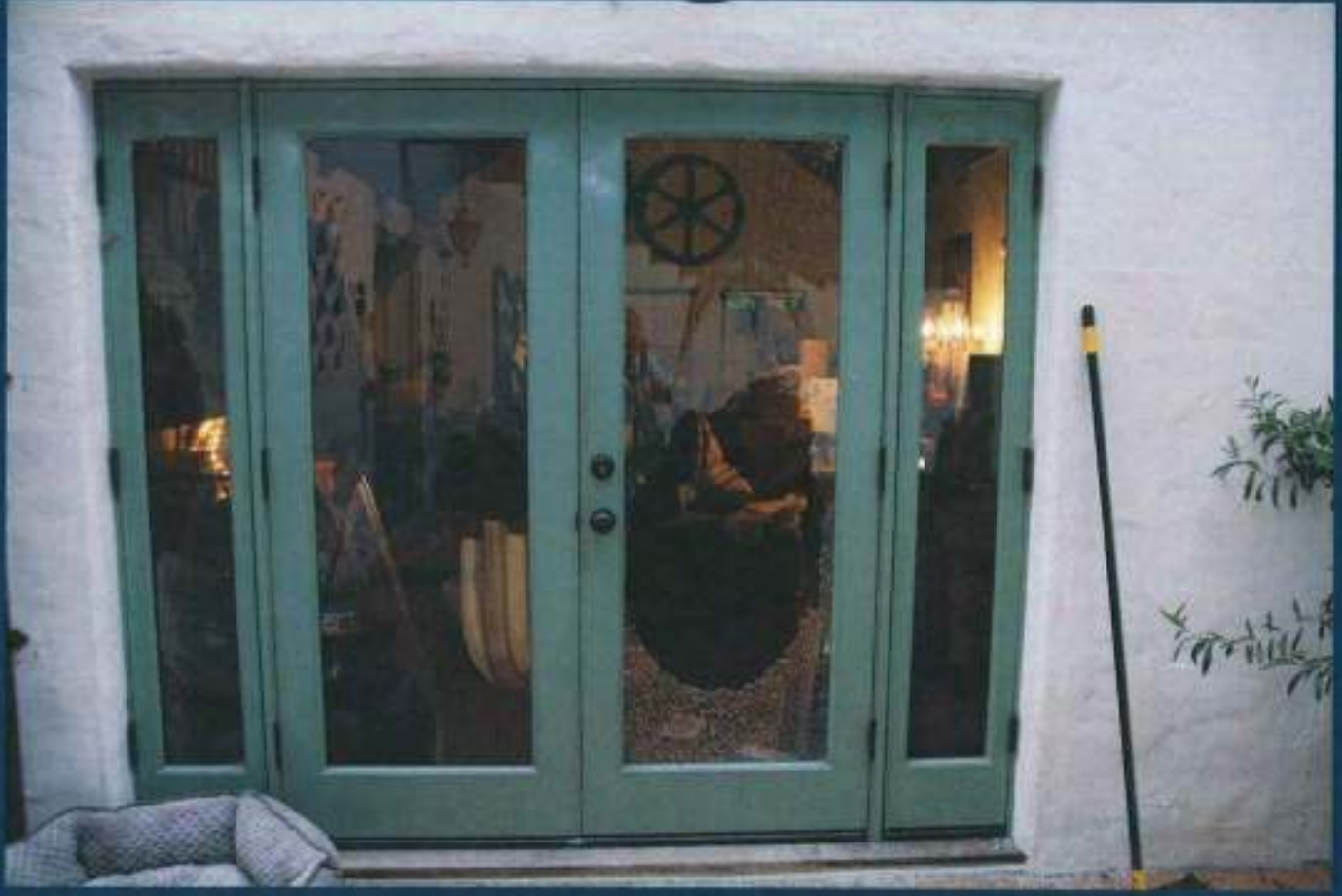
Point of Entry
